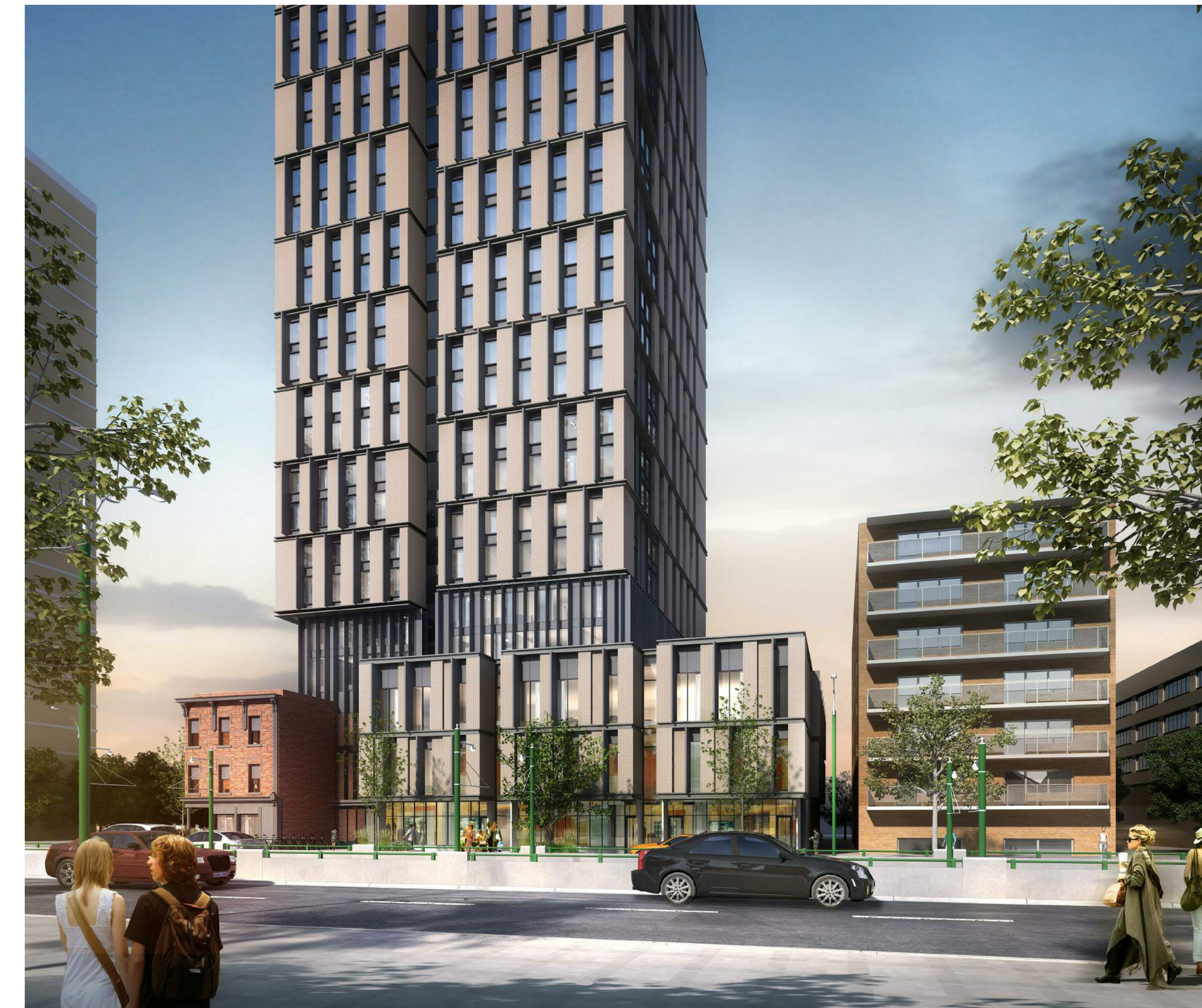
EAST FACADE ON SPADINA
