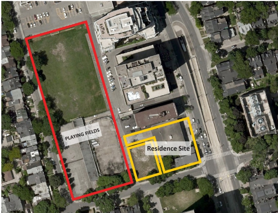
Figure 1.2 Existing Site Aerial
