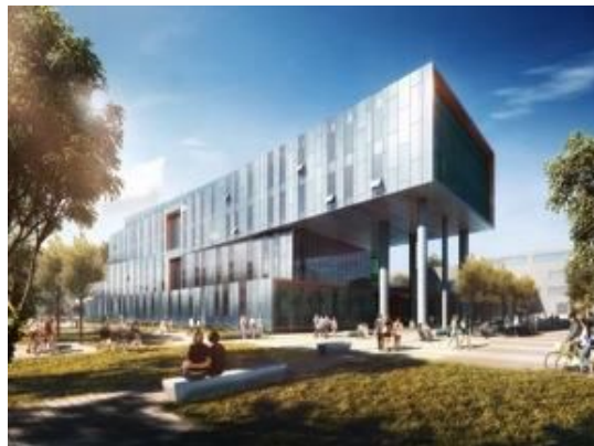
View from Military Trail (North West Corner)
