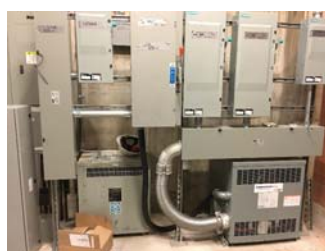
New electrical conduits from CUP to labs
