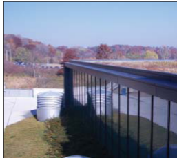
Green Roof, RAWC Building
