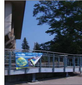
Accessible Entry, Davis Building
