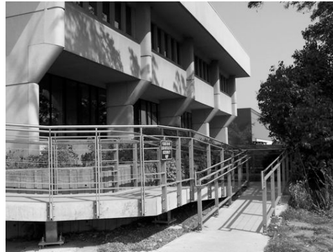
Existing exterior view – SW Entrance
