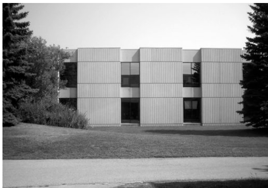
Existing exterior view – NW Elevation
