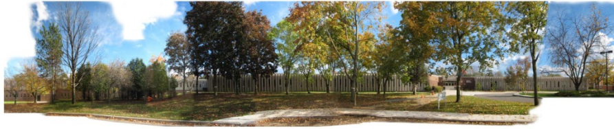
View of North Building's west facade with entrance drop-off in foreground
