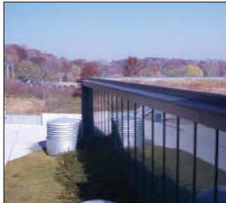
Green Roof, RAWC Building
