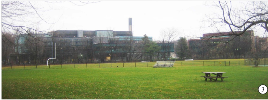
View of athletic field (future Campus Green) and Instructional Centre under construction
