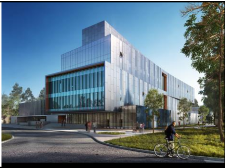
VIEW FROM NORTH
