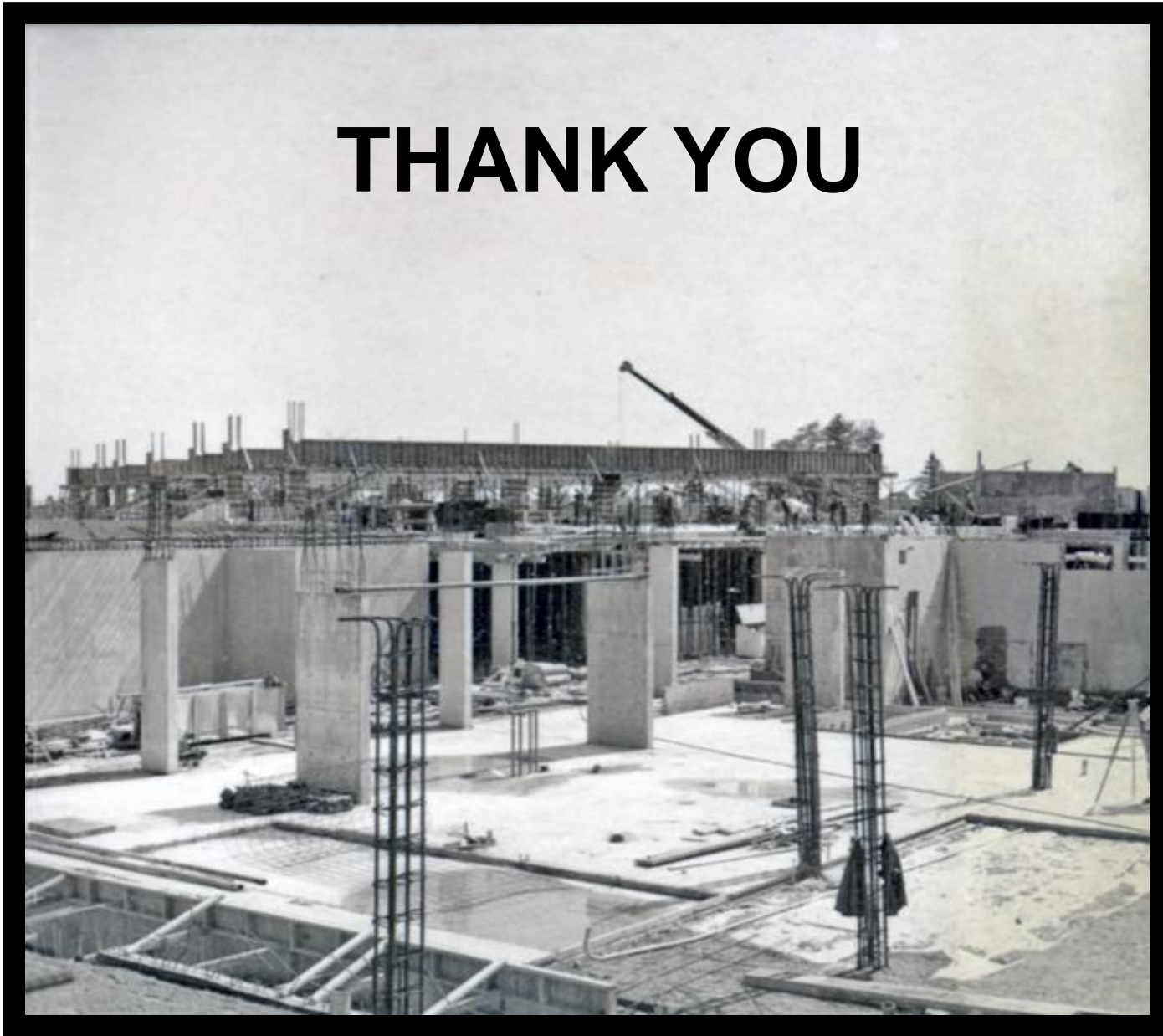
The Original, "Temporary" North Building Under Construction
