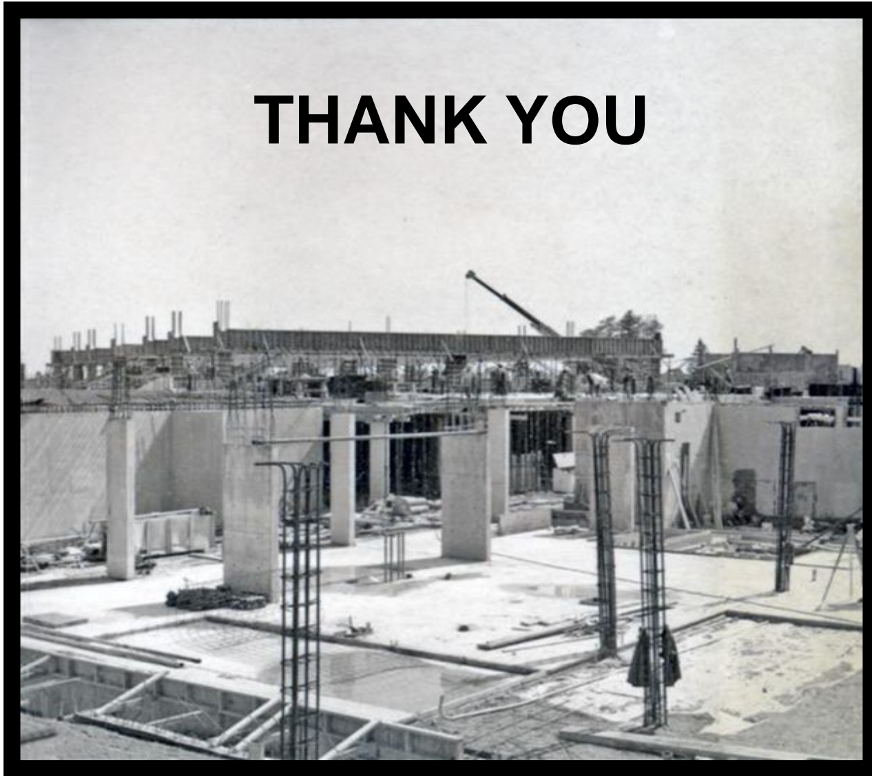
The Original, “Temporary” North Building Under Construction
