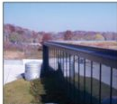
Green Roof, RAVC Building
