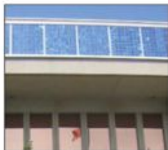
Solar Panel Array, Davis Building
