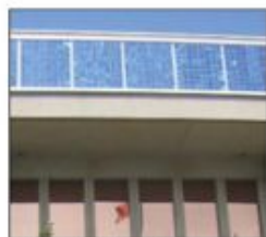
Solar Panel Array, Davis Building The solar panel retrofit on the Davis Building is a prominently displayed example of a sustainable energy technology in use at UTM. Displays inside the building provide real-time energy use data.
