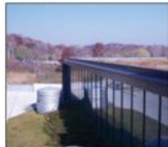
Green Roof, RAVC Building The green roof on the RAVC facility is an example of sustainable building technology that mitigates storm water run off, provides additional habitat for local species, and reduces both building cooling loads and the campus' urban heat island effect.
