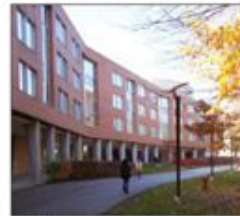
Erindale Hall, north elevation
