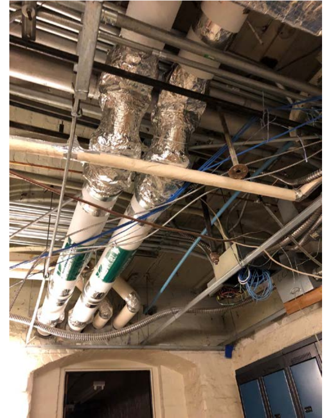
Convoluting piping around existing pipes.
