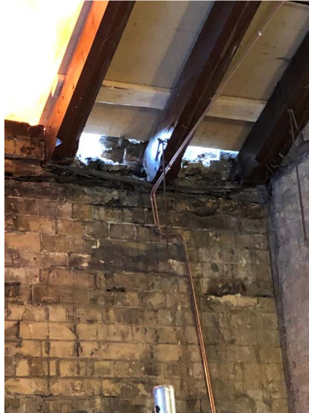
Roofing condition at the top of the planned elevator
