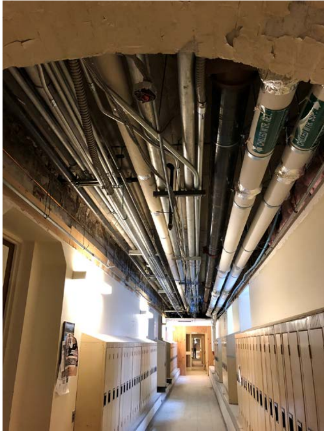
As-built drawings showed only one pipe
