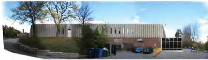
North Building service entry at the south of the site
