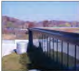
Green Roof, RAWC Building
