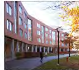
Erindale Hall, north elevation
