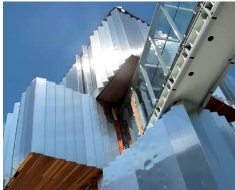
The Terrence Donnelly Health Sciences Complex houses the Mississauga Academy of Medicine. The academy delivers programs in health sciences to more than 200 students every year.
