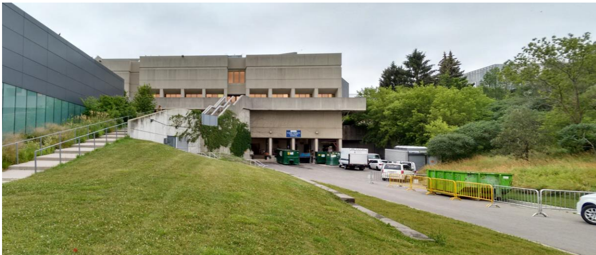
View from Outer Circle Road, towards west, Davis Building Loading Dock, Site 1 at right.
