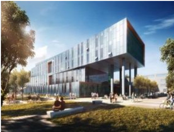
View from Military Trail (North West Corner)
