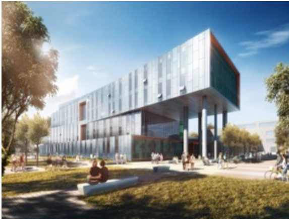
View from Military Trail (North West Corner)
