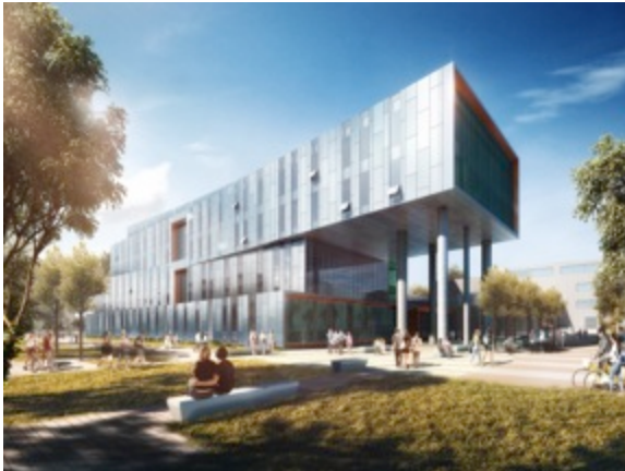
View from Military Trail (North West Corner)
