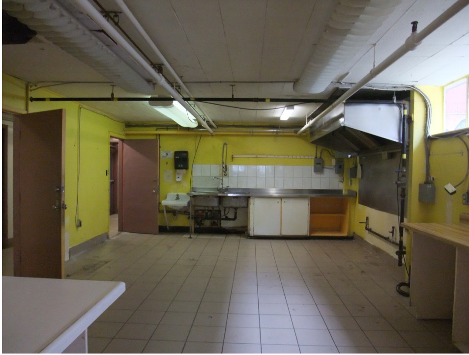
167 College Street, Basement Kitchen, Existing
