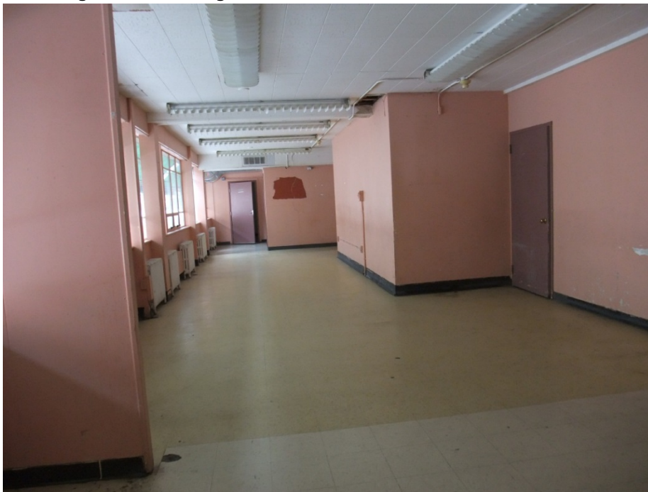
167 College Street, Ground Floor Lounge, Existing
