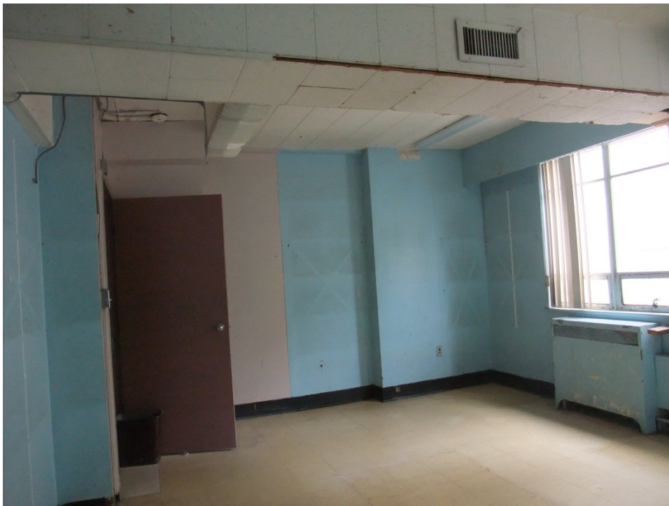
167 College Street, Ground Floor Dorm, Existing
