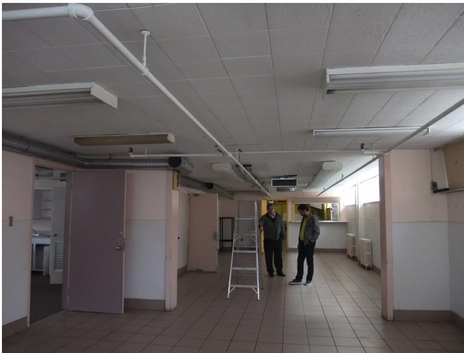
167 College Street, Basement Dining Hall, Existing
