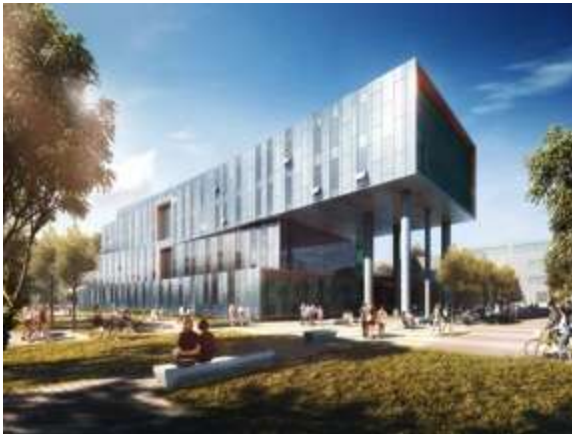
View from Military Trail (North West Corner)
