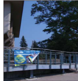
Accessible Entry, Davis Building
