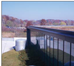
Green Roof, RAWC Building
