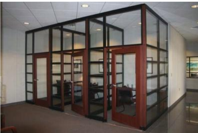
Figure 15. Example of private office with glass walls.
