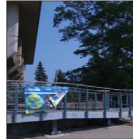
Accessible Entry, Davis Building
