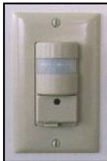
Infra-red sensor detects occupancy.
