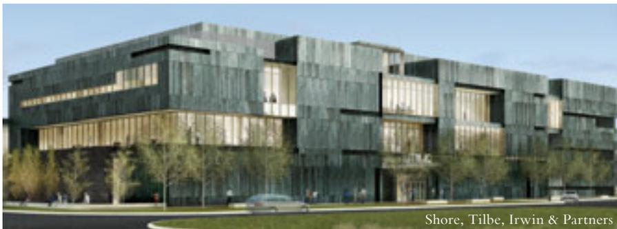
Above: University of Toronto Mississauga's new Instructional Centre will use energy and water-efficient fixtures, as well as local materials with renewable or recycled content, and will include a green roof. Geothermal pipes will help regulate the temperature inside the building all year round.
