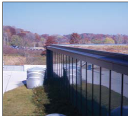
Green Roof, RAWC Building
