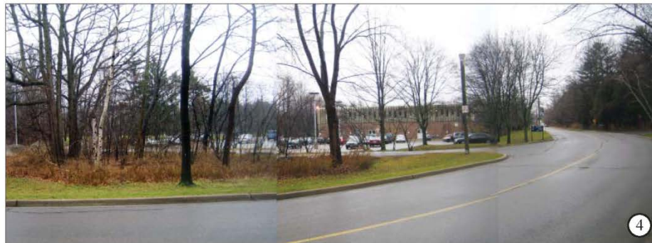
View from Outer Circle Road toward parking Lot 1 and the North Building
