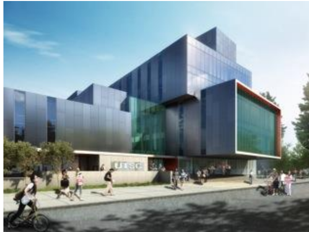
East Entrance Facing Transit Loop (South East Corner)
